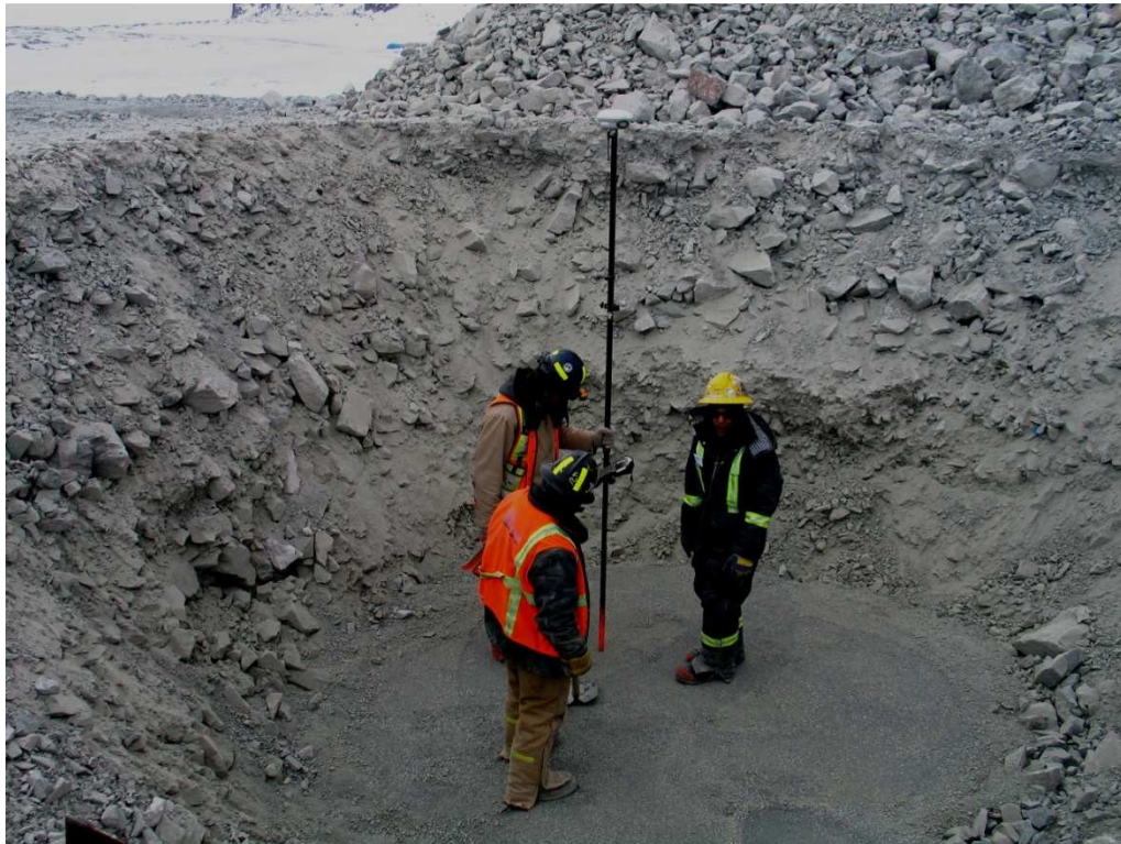
Photo 10: Survey check before survey monument installed. Crush bedding has been packed. ND-SMP-100-US
