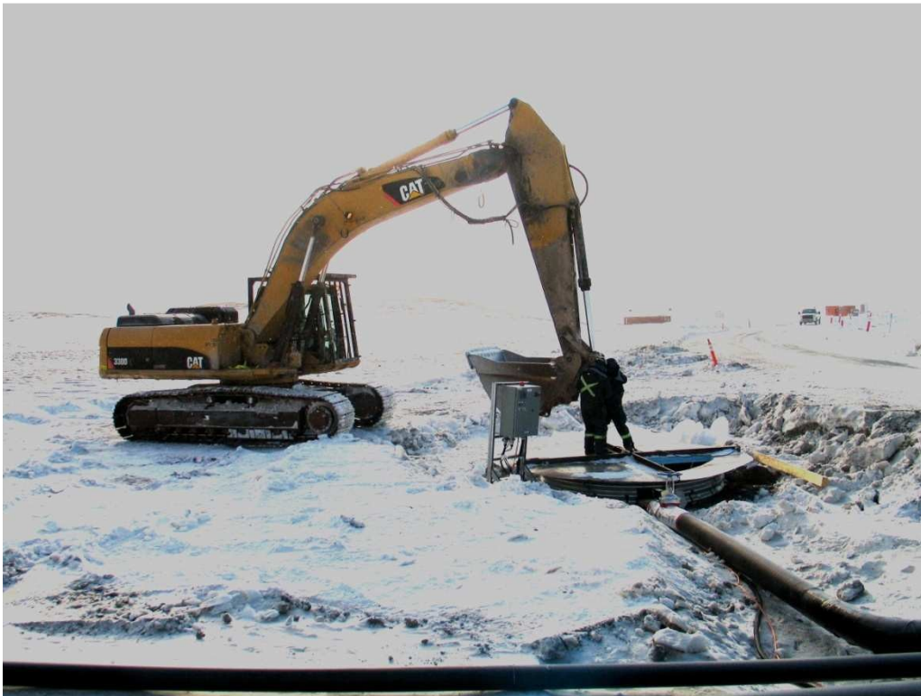
Photo 1: Installation of sump lid at Sump 2.
