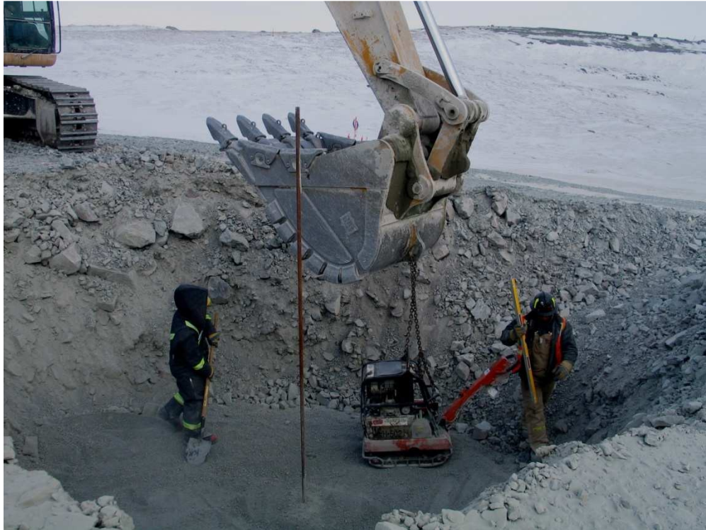
Photo 11: Moving packer into place. Crush over plate. ND-SMP-100-US
