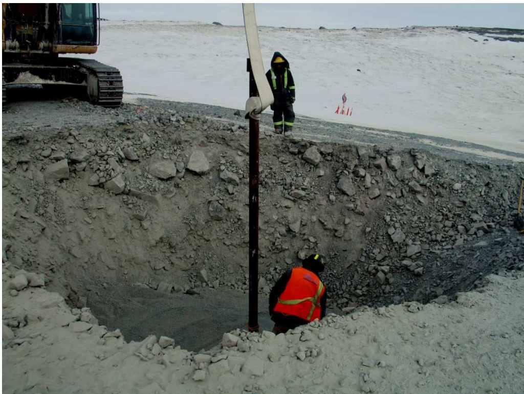
Photo 12: Setting pipe in place. ND-SMP-100-US.
