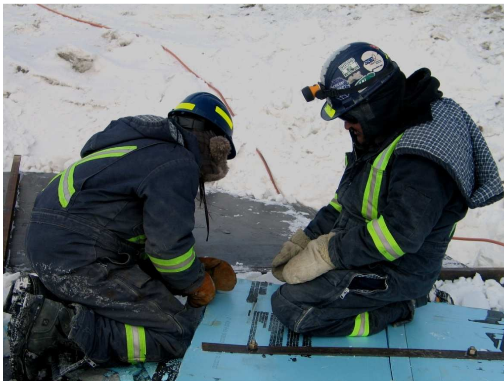
Photo 5: Trimming insulation on access panel to get panel to fit..
