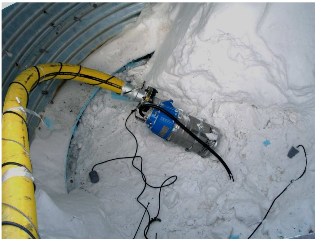
Photo 3: Submersible pump in Sump 1.
